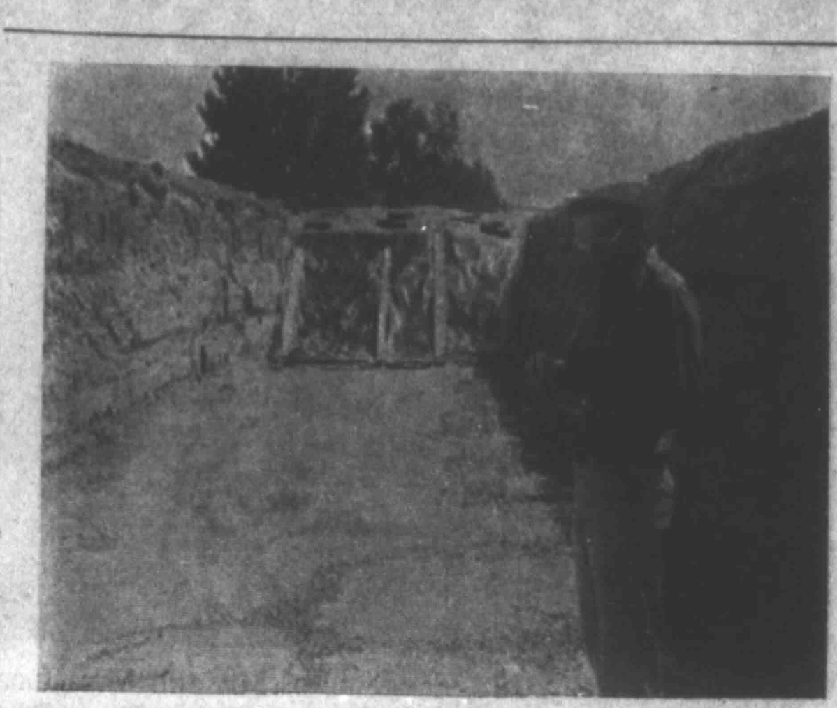
HARRY WRIGHT, Jr., of Halls, examines silage from his newly built trench silo—175 feet long, 14 feet across the bottom, 20 feet across the top, nine feet deep. A concrete floor aids handling of the more than 500-ton capacity, high quality feed to supplement winter pasture for his beef herd.
